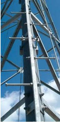
Welded Sections used on sections #13-21
